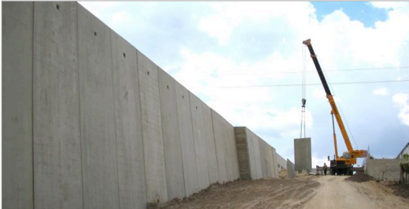
FAIR-FACED CONCRETE WALL
