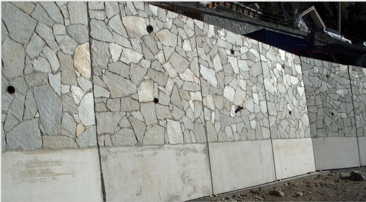
FAIR-FACED CONCRETE WALL
