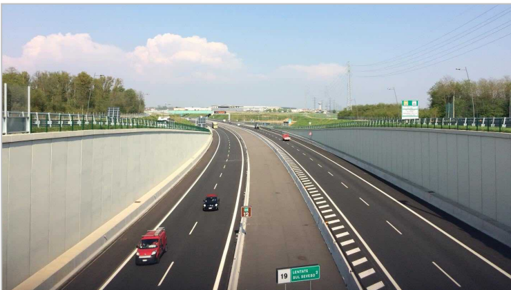
FAIR-FACED CONCRETE WALL
